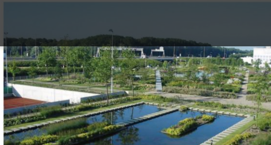
European Patent Office, Rijswijk, NL | The 25,000m 2 roof garden includes a series of gardens including a wetland and lake with ecological value | Photo: Copijn Tuin- en Landschapsarchitecten
